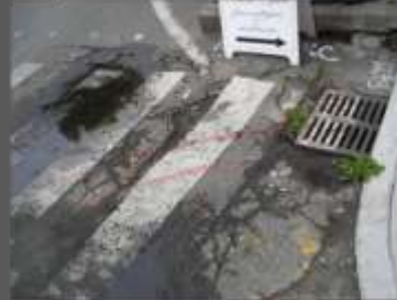
Asphalt Cracking
