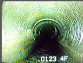
Fractured/Broken Pipes
